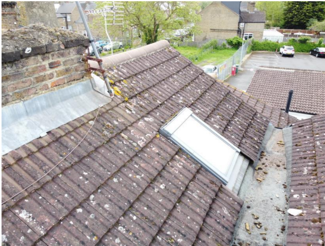
V- Lux style window appears to be blocked up from the inside
